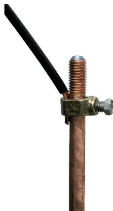
FIGURE 5-14. The #4 cable connected to the ground rod
